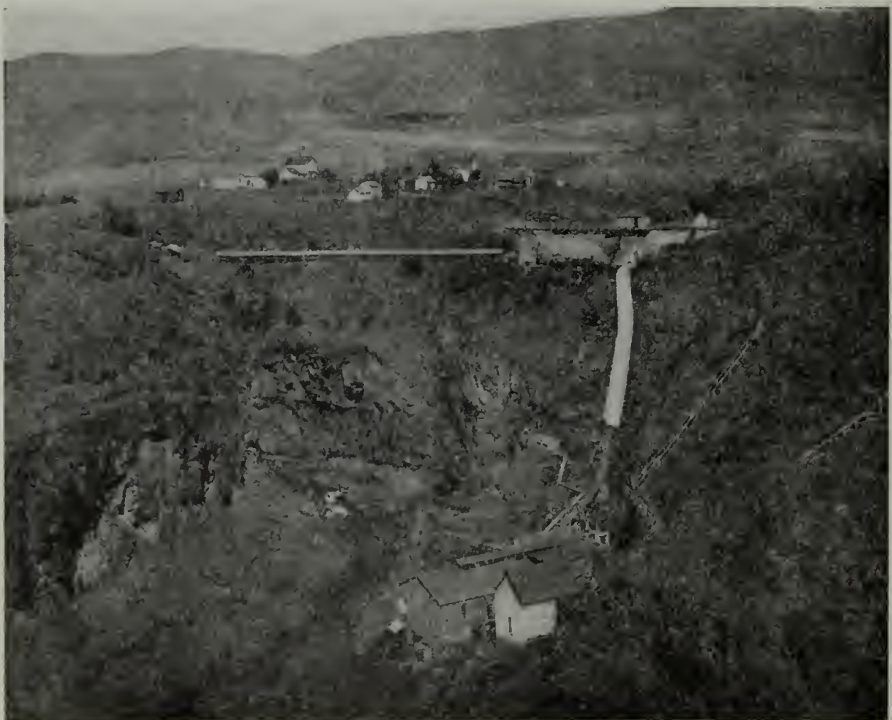
Tygh Valley Generating Station - as it appeared December 31, 1936.
